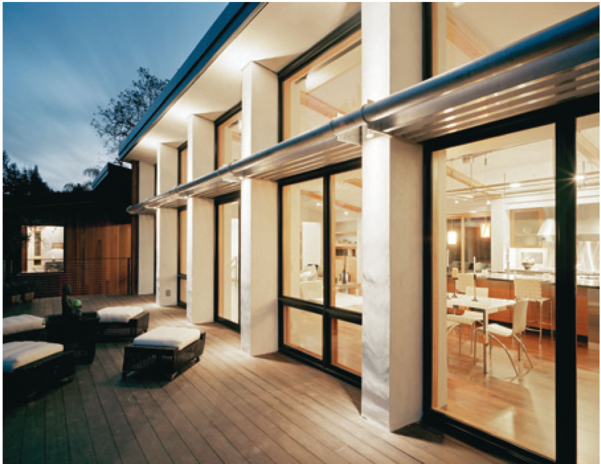
Jones Residence/Redwood City, California, photos by Mark Trousdale
